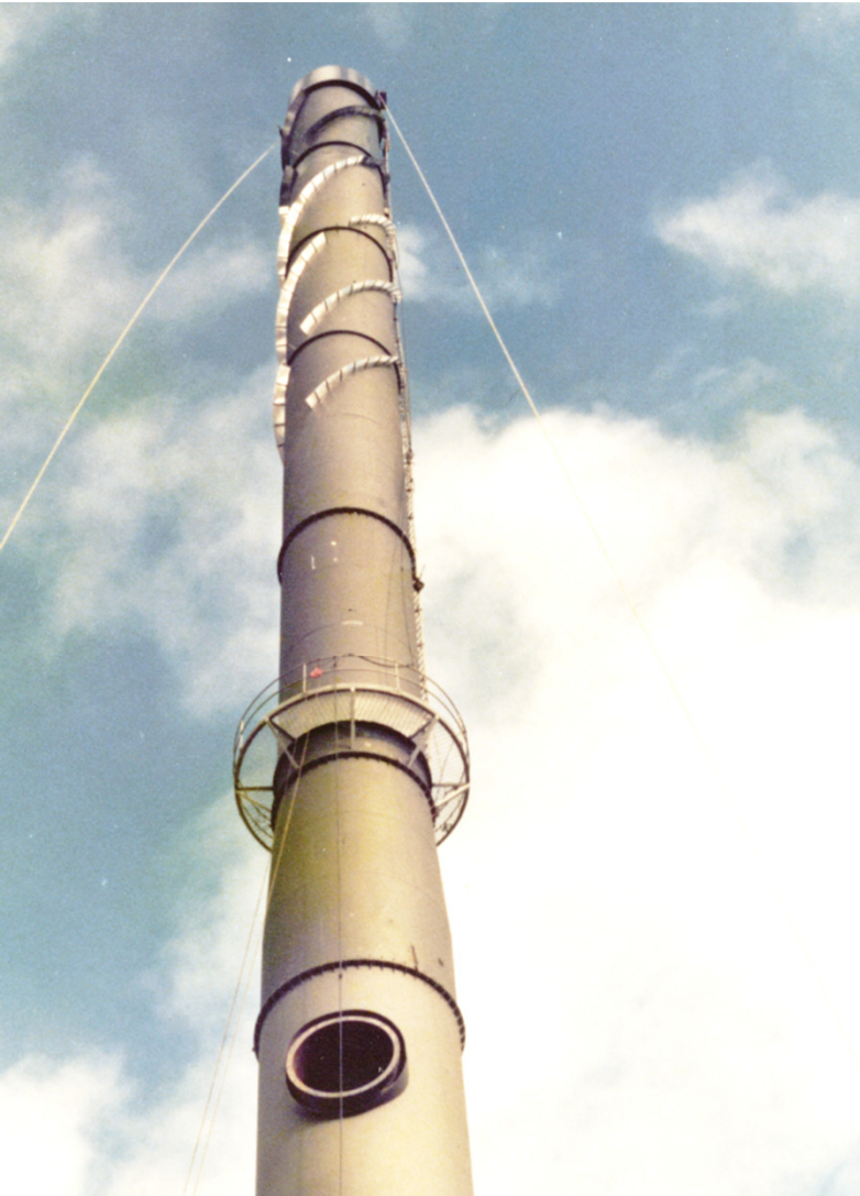
Vibration stack with helical strake temporary stabilized with cables
